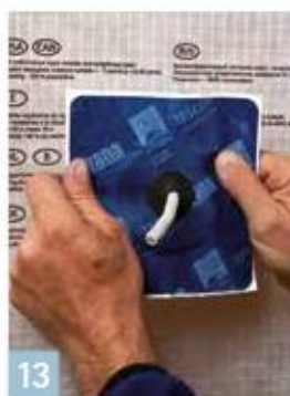
13 Joints to pipes and cables
