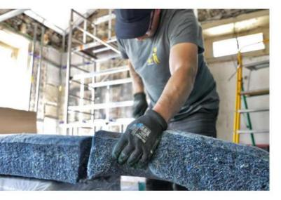
The COTONWOOL FLEX 25 process is the subject of a Technical Appraisal (no. 20/19-439\_V2 wall application, 20/19-440\_V2 loft application). It is designed for thermal insulation in new build and renovation work on the following buildings:
